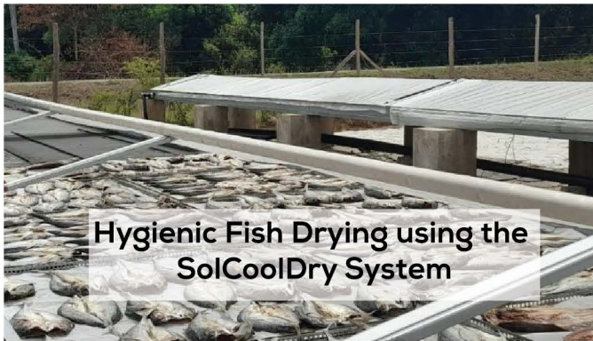
SolCoolDry System installed at Mwazaro, Kwale County.
